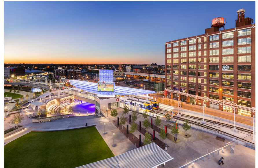
Target Field Station, Minneapolis, MN
