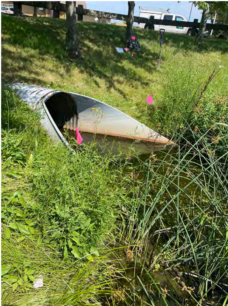
Photo 38 – South end of the culvert connecting the two sections of Wetland NFB W-3.
