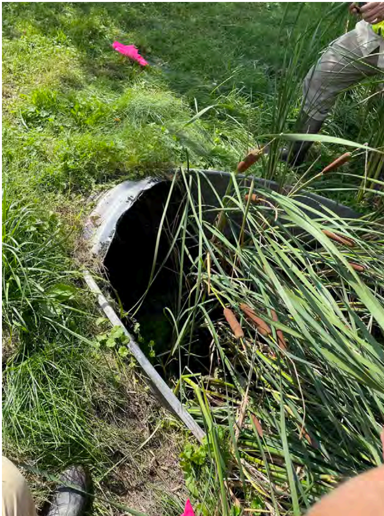
Photo 39 – North end of the culvert connecting the two sections of Wetland NFB W-3.
