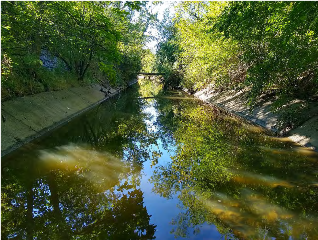
Photo 2 – Bizer Creek south of Rensch Road. The channel width at water level was 19.0 feet on July 20, 2021. The width of the top of the concrete channel is 26.2 feet.
