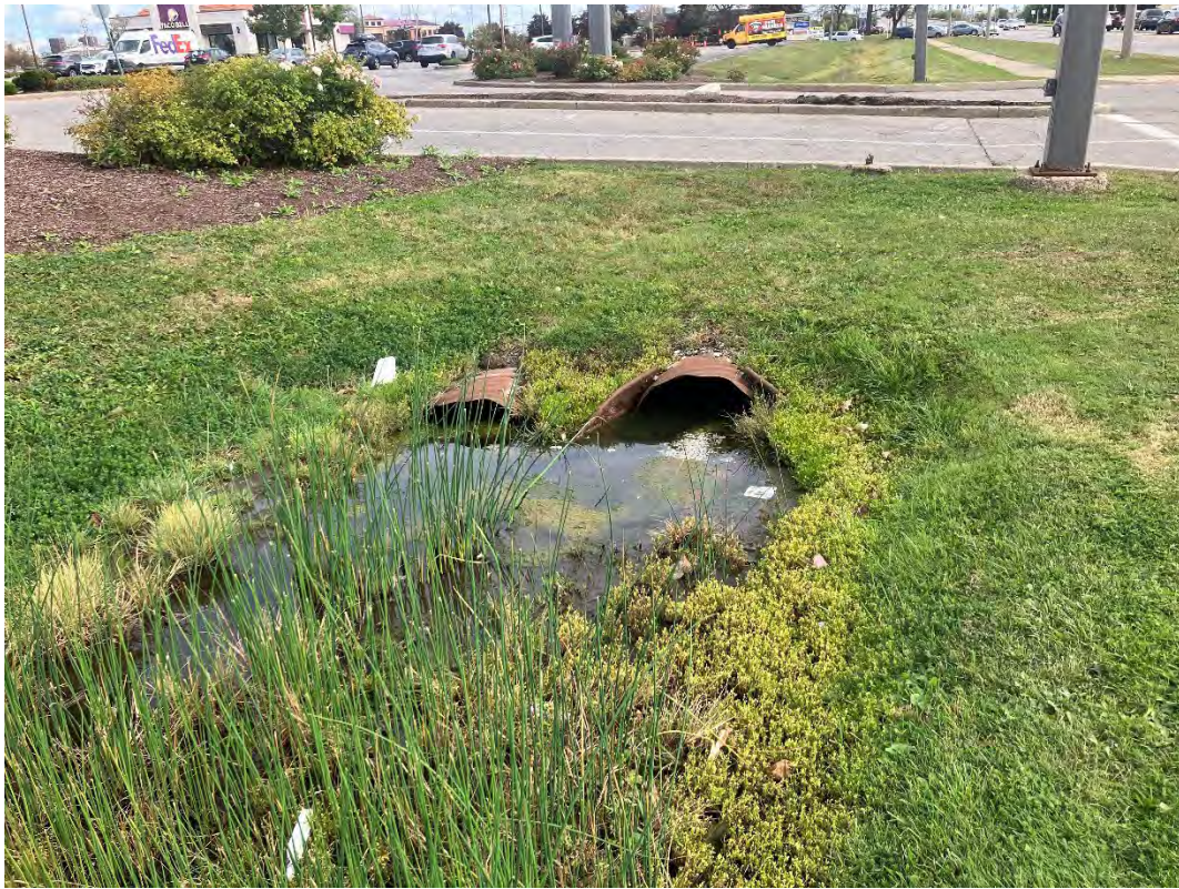
Photo 45 – Culverts connecting the eastern and western sections of Wetland MR W-1.
