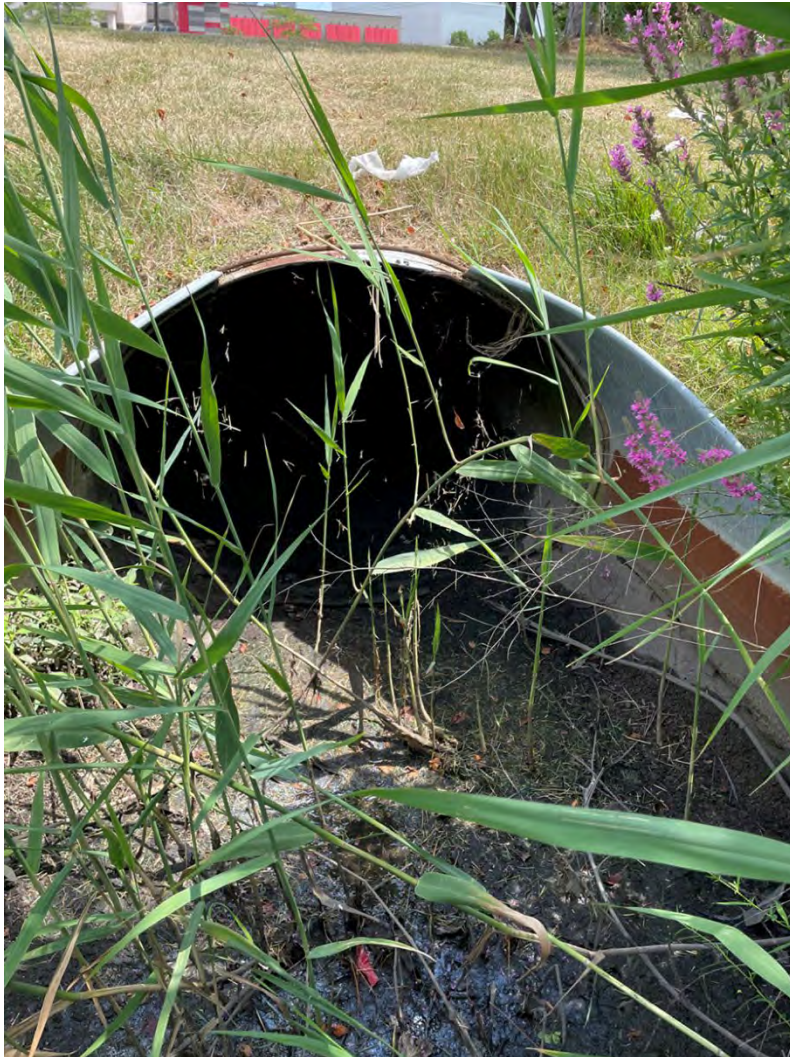
Photo 32 – Large culvert that drains Wetland NFB W-2. Water flows under the mall parking lot east of Niagara Falls Boulevard and South of Maple Road.
