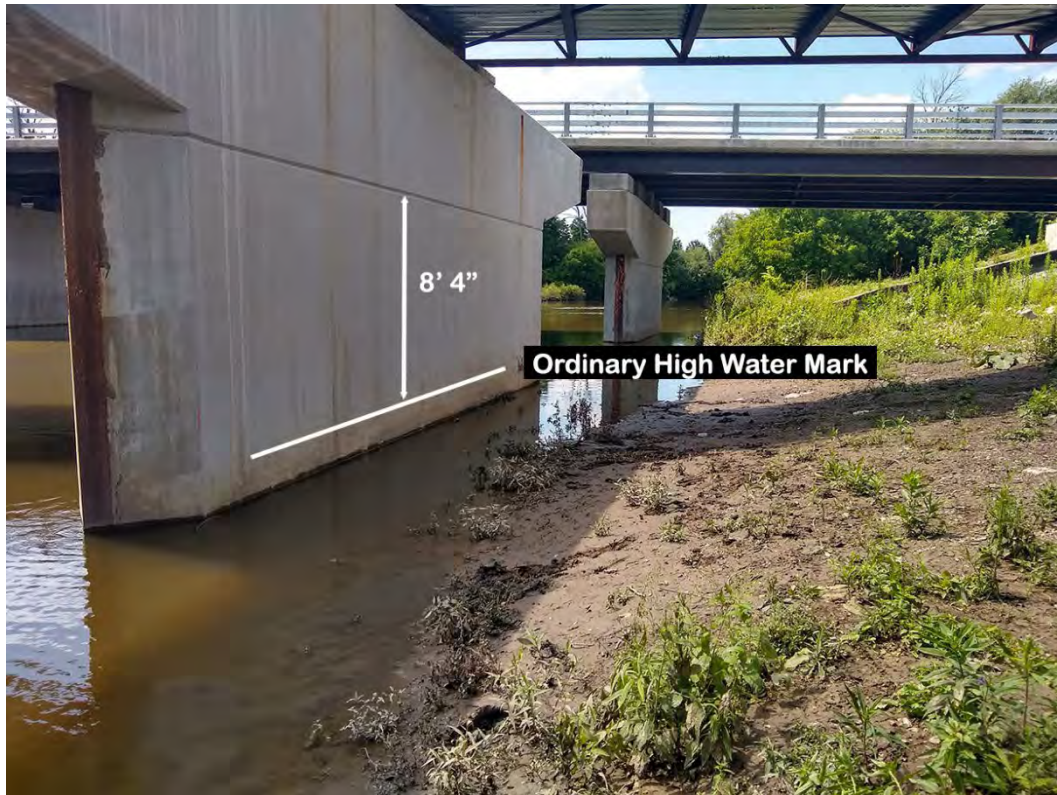
Photo 9 – Ordinary high water mark (OHWM) of Ellicott Creek on the northeastern pier of the bridge for the pedestrian/bike trail adjacent to the John James Audubon Parkway Bridge. The OHWM is 2.0 feet above the stream bed at this location.
