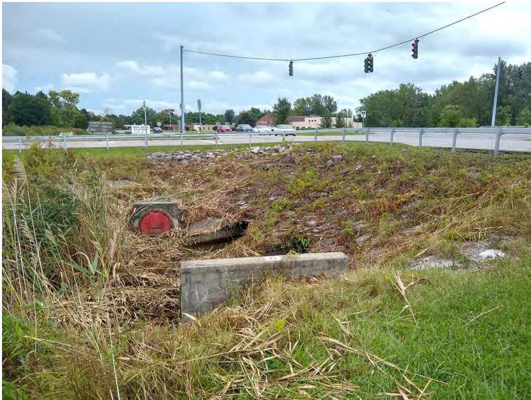
Photo 18 – The west end of Wetland JJA W-4 looking south toward Wetlands JJA W-2 and JJA W-3.
