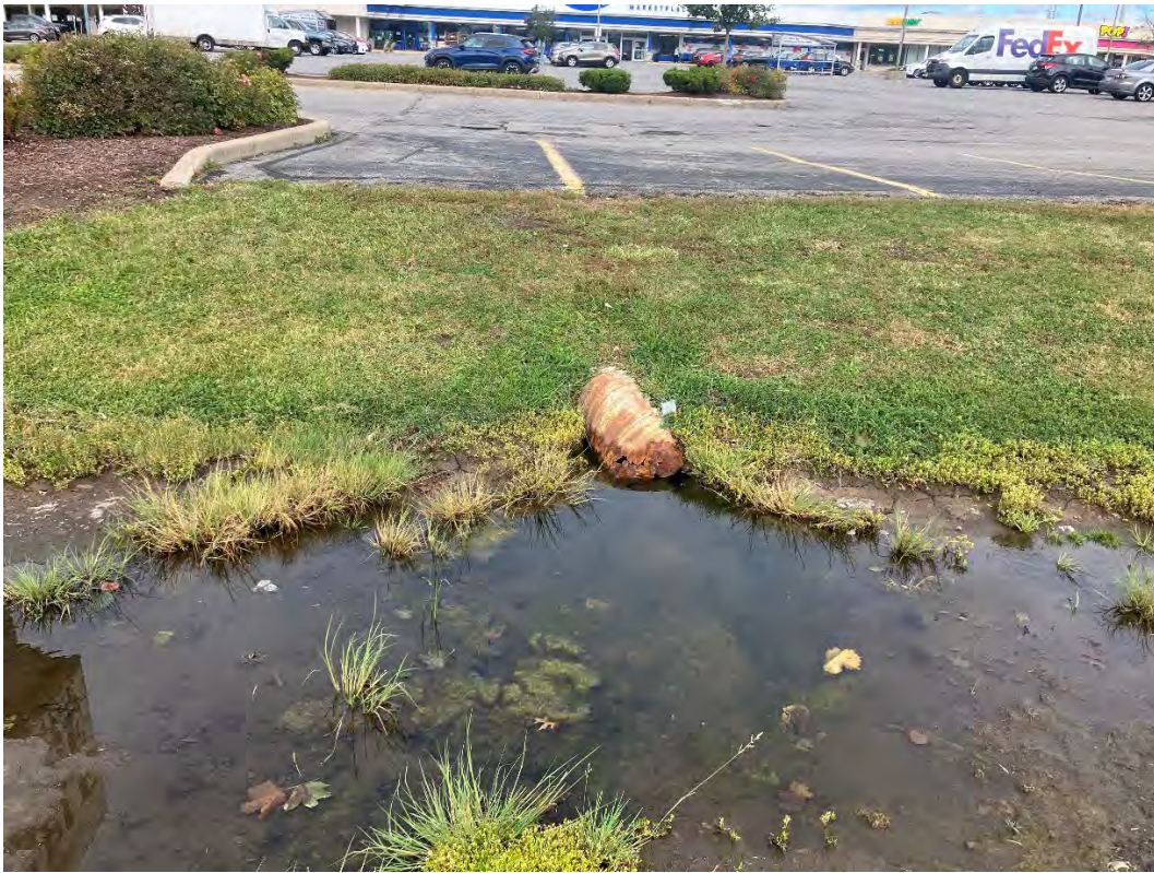
Photo 46 – Multiple culverts drain the parking lot north of Wetland MR W-1.
